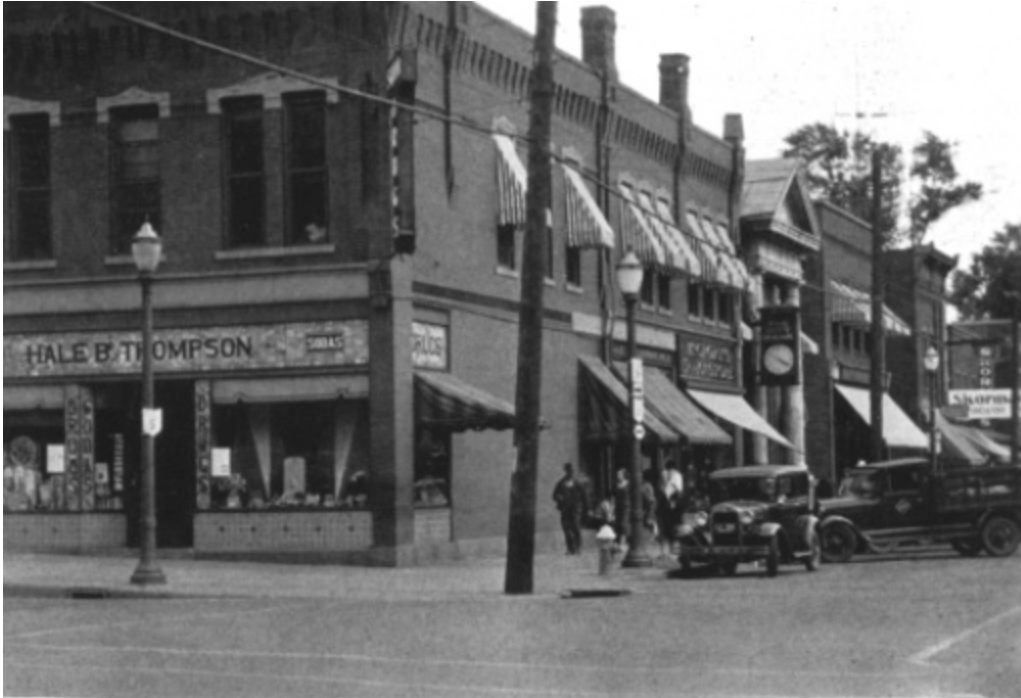
Looking south on Water Street from Main Street
